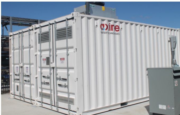
Axine's on-site system installation
