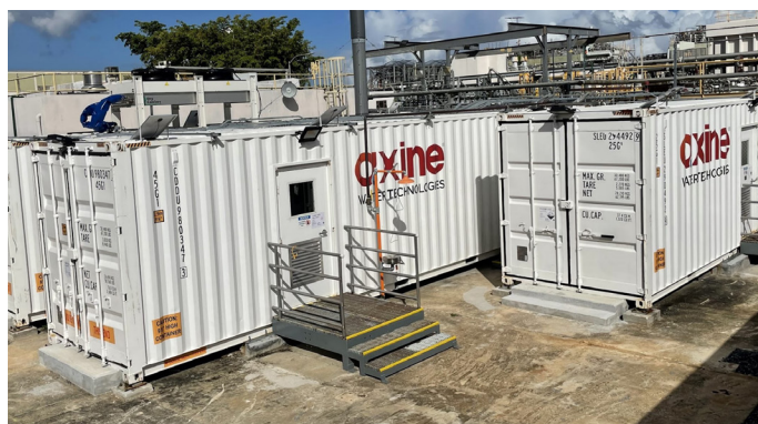
Axine's on-site system installation
